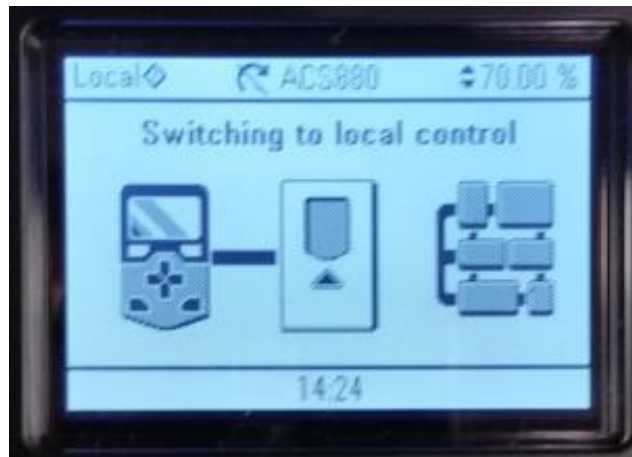
Figure 14: VFD Interface Depicting Switching from Remote to Local Mode
